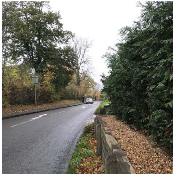
Photo 2. Sight line for pedestrian attempting to exit from 37 Hare Lane (note absence of footpath), shorter still in a car
